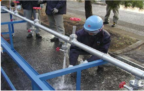
Remove the sediment of the clogged drain valve using a wire
